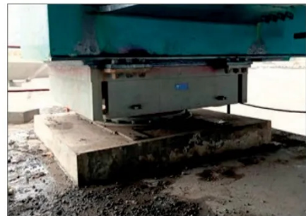
Fig. 14: Installed bearings
