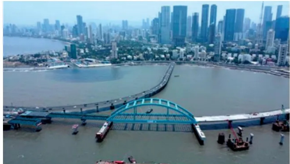
Fig. 2: Arch bridges, MCRP
