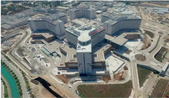
Fig. 6 The Adana City Hospital in Turkey with a seismic isolation system helped it to stay up and functioning during and after the earthquake (Source: Ref.13)
