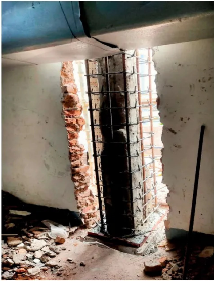
Fig. 3: Concrete Jacketing of Column
