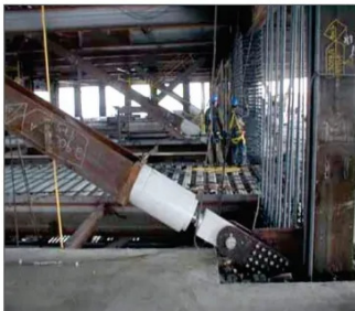
Fig.4: Damper installation
